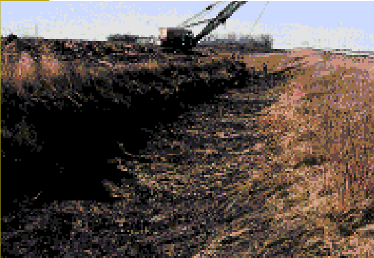
Wetland drainage in North Dakota.
