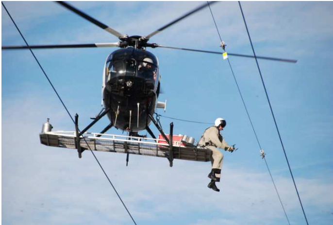
Crew replacing bird flight diverters on Rowe Sanctuary
