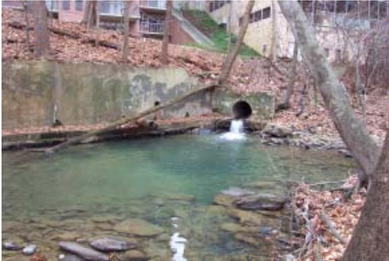
Another view of the outfall discharging into Soapstone Creek behind 4411 Connecticut Avenue, NW. Note also the other outfalls, and the discoloration of the water.
